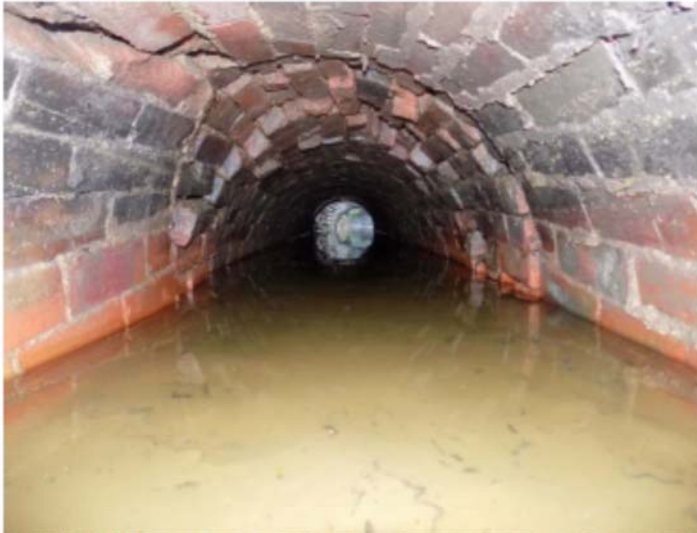
Park Drain Culvert, Thorganby
