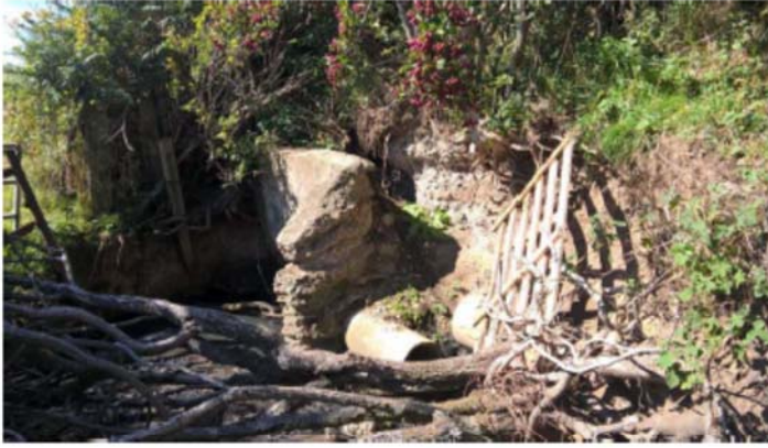
A170 Valley View Culvert
