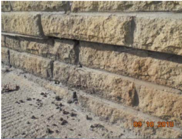
Retaining Wall Foreshore Road, Scarborough;
